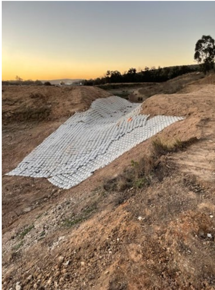
Figure 6: Earthlok installation on the inlet of SD17 (LDP 1)
