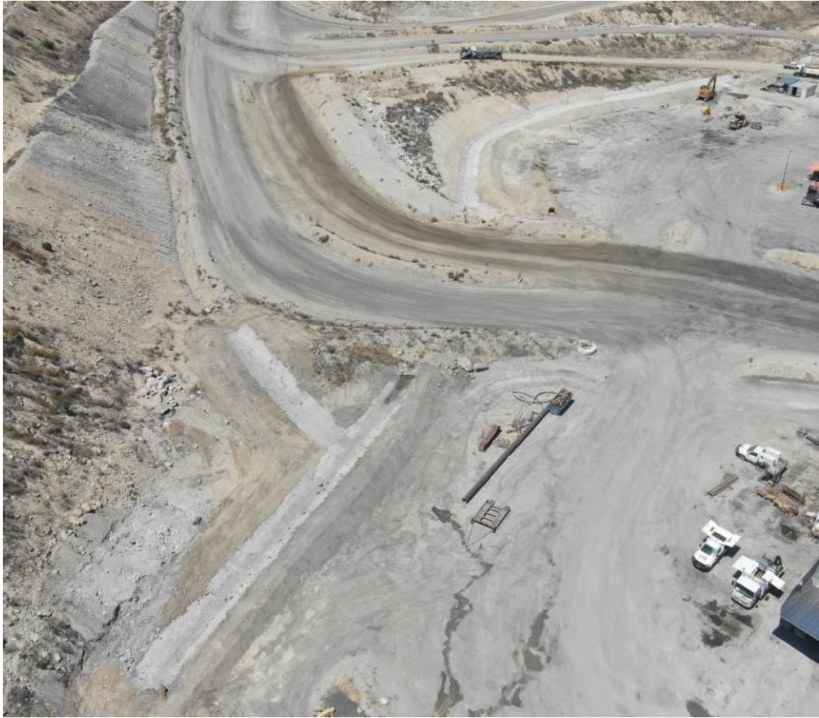
Figure 5: Earthlok installation on the drain from the ROM pad to SB16A
