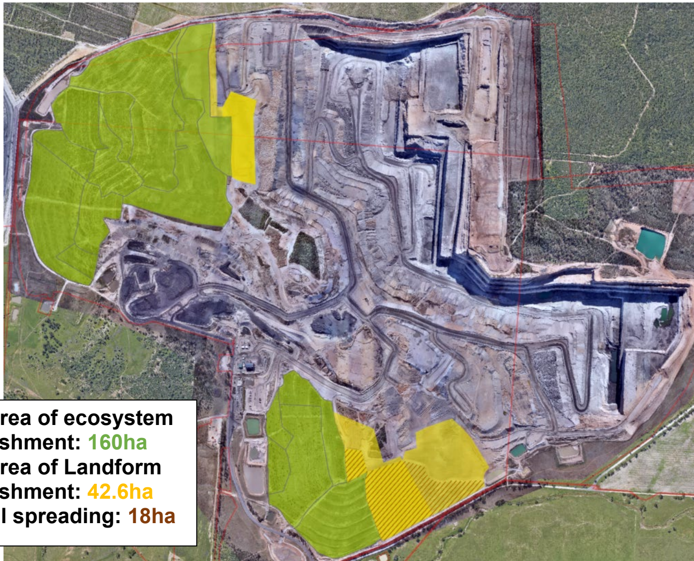
Figure 5: Rehab Status as at end of July 2023
